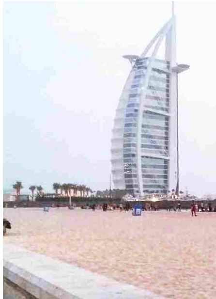
Figure 2: Burj Al Arab – Exterior view (Source: Author, 2015)
